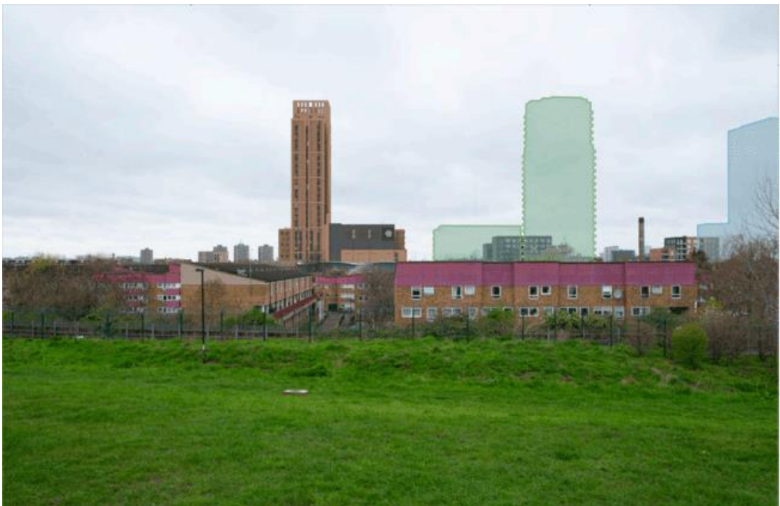
Image 31 (above): Verified view across Bridgehouse Meadows in the proposed scenario, showing the proposed development (in full render) in the centreground, the development at 227-255 Ilderton Road (known as Leatham scheme) which is under construction (in green) and the Ilderton Wharf scheme (in blue)
